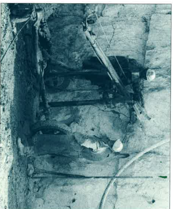
Bottom hole drilling 1951.
