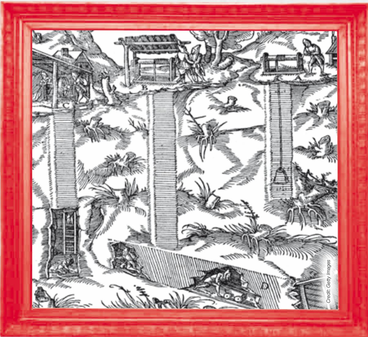
► Illustration of a sectional view of a mine, taken from Agricola's *De Re Metallica*, published in 1556.
